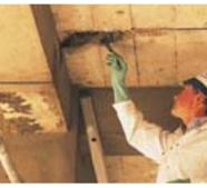
Restoring Profile. CRS REPAIR MORTAR HB. High-build repair mortar ideal for overhead application.
