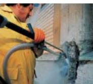
Remove rust and clean reinforcement steel by sandblasting or other suitable mechanical methods.
