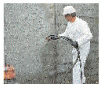
Surface Levelling. CRS LEVELLING COMPOUND LC is used for surface levelling over the CRS repair and surrounding concrete. Also provides an ideal substrate for the protective coating.
