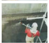
If available use highest waterpressure technology and remove unsound concrete completely. Expose corroded reinforcing steel. Remove rust and clean.
