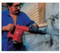
Carefully remove unsound concrete and expose reinforcing steel completely.
